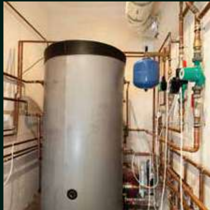
RAINWATER HARVESTING SYSTEM
