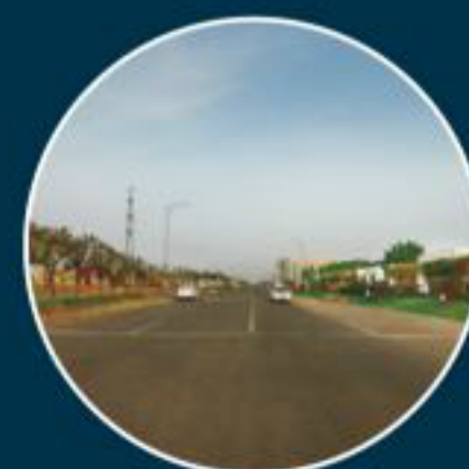
WELL DEVELOPED SECTOR ROADS FOR INTERNAL CONNECTIVITY
